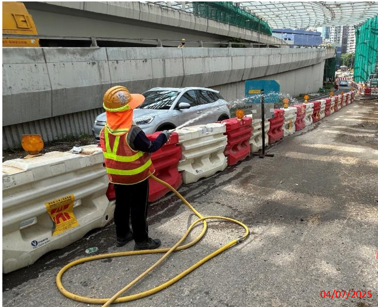
Remark 2: Site photo of dust mitigation measure
